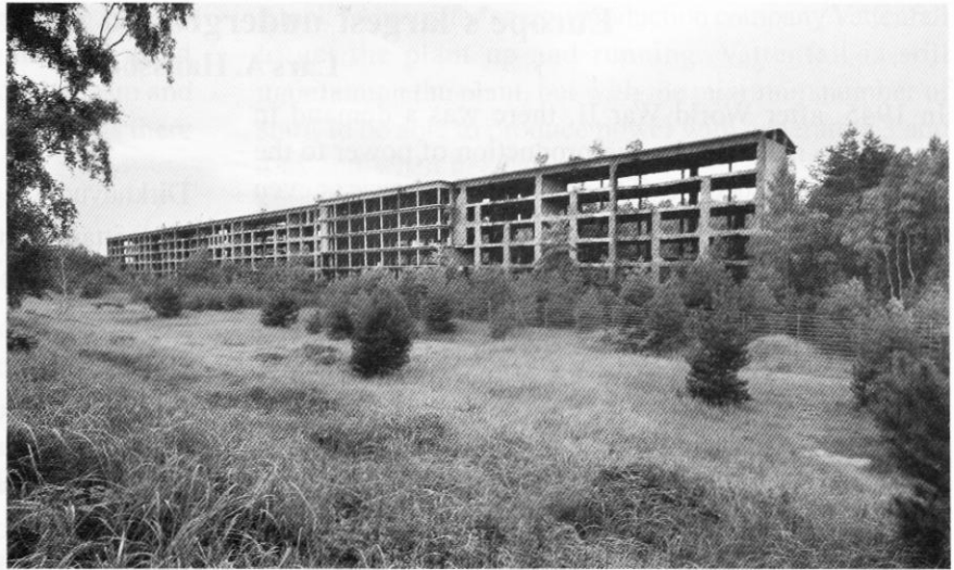
At the north end of the complex some blocks have been demolished while others have been partly demolished and are now in a dangerous condition
